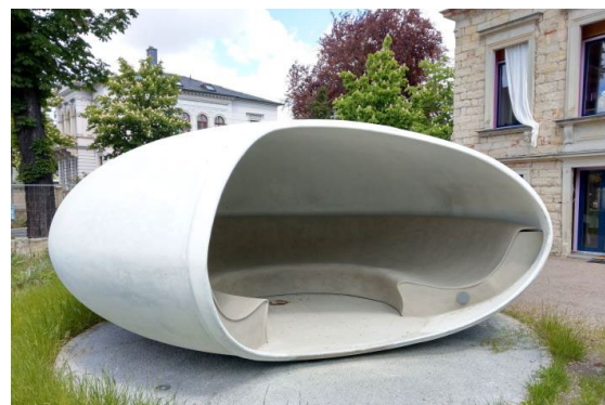
Fig. 3: "Smartie" made of textile reinforced concrete
