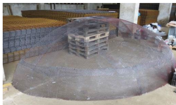
Fig. 2: Filigree reinforcement made of carbon fibers
