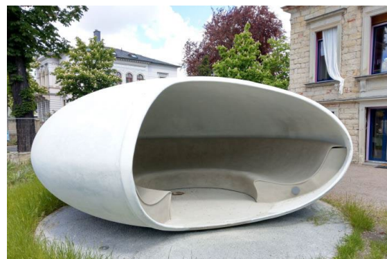
Fig. 3: "Smartie" made of textile reinforced concrete
